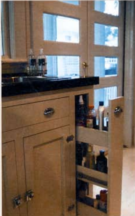
Gilbert noticed the carpenter was going to fill in this space with wood, but he suggested, instead, that it might be a great pullout drawer for cleansers.
