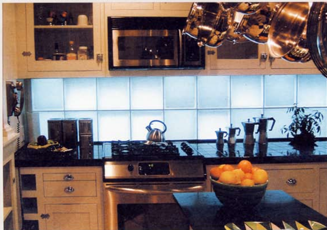
Gilbert bought for $5 apiece translucent glass blocks that once were in the former Gulf Publishing Building. He picked out 20 of the best looking—the ones with the fewest nicks—and constructed a backsplash that allows outside light to filter through.
